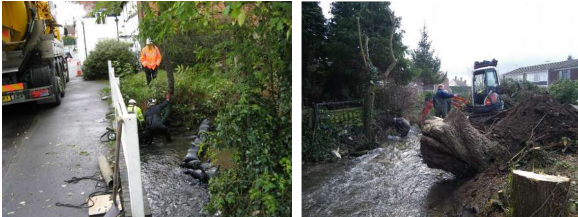
Flood prevention work at Grove
